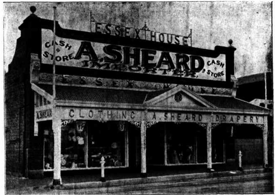
ESSEX HOUSE (NEW BUILDING).
