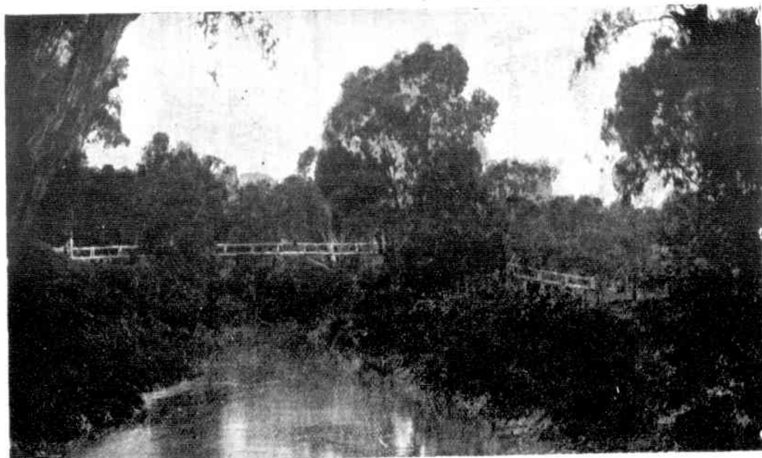
GOOSE ISLAND BRIDGE, GAWLER, S.A.
